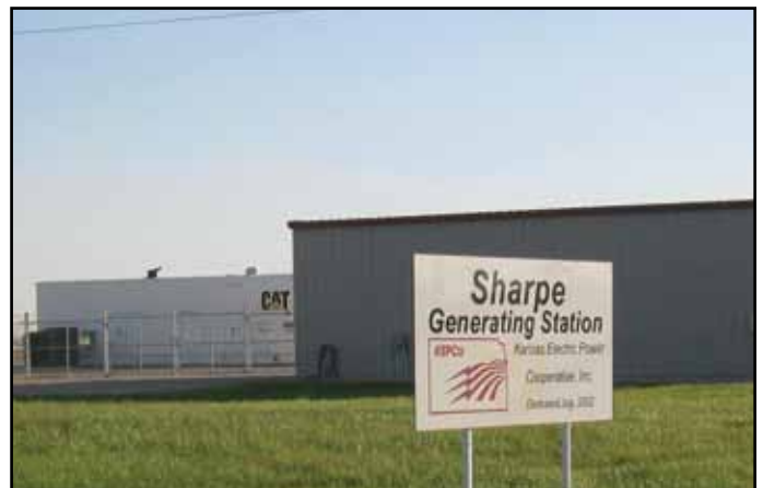
Sharpe Generating Station Diesel Peaking In Service, June, 2002 20 MW
