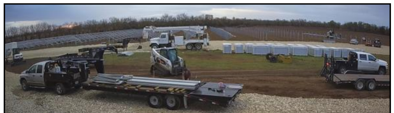
Delivery of materials
