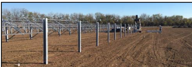
Piles ready for installation
